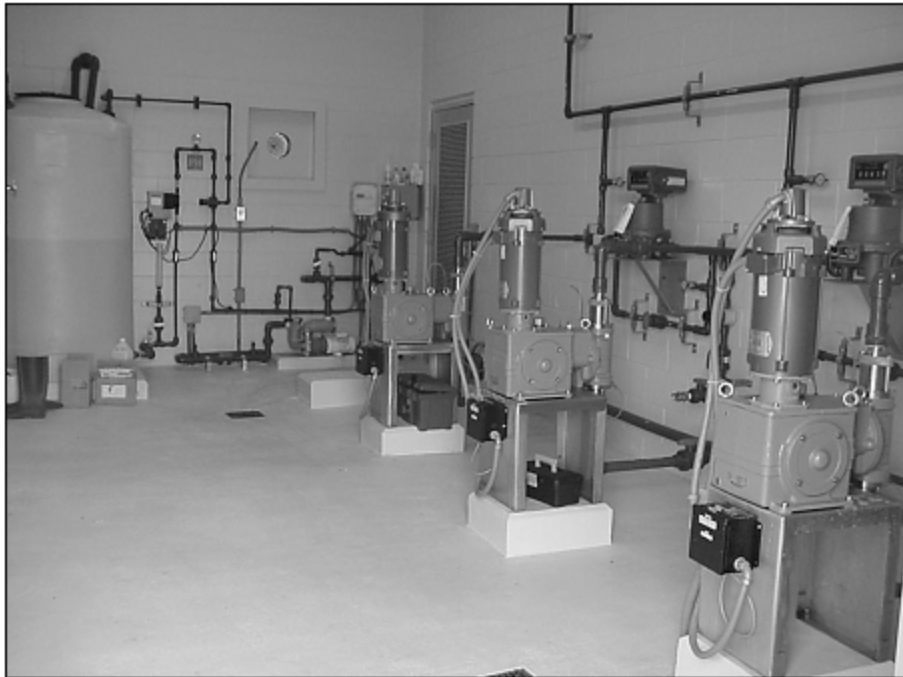
Figure 3.3.9-1. Alum Treatment System and Injection Equipment
