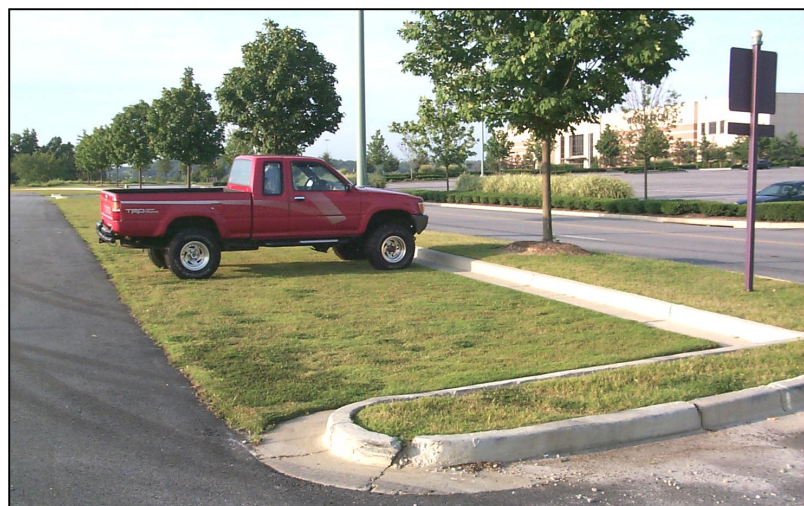
Figure 1.4.2-21 Grass Paver Surface Used for Parking
