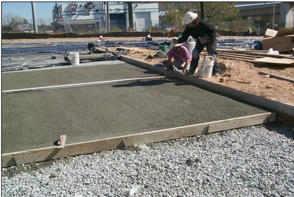
Figure 3.3.7-2 Porous Concrete System Installation
