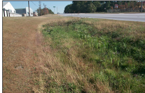
Enhanced Wet Swale
