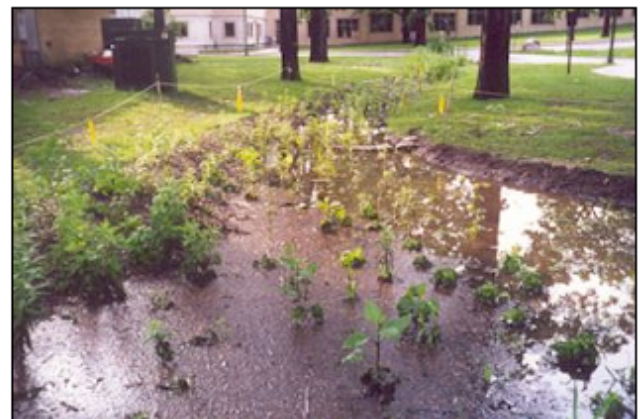
Newly Planted Bioretention Area After Storm
