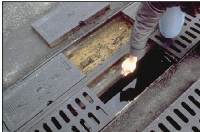
Perimeter Sand Filter
