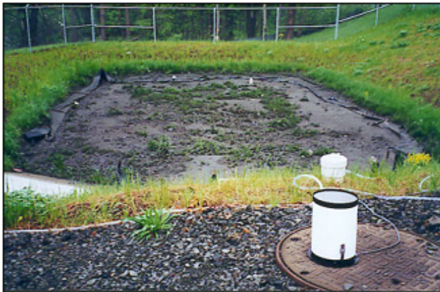
Surface Sand Filter
