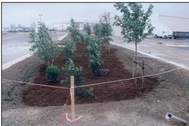
Newly Constructed Bioretention Area
