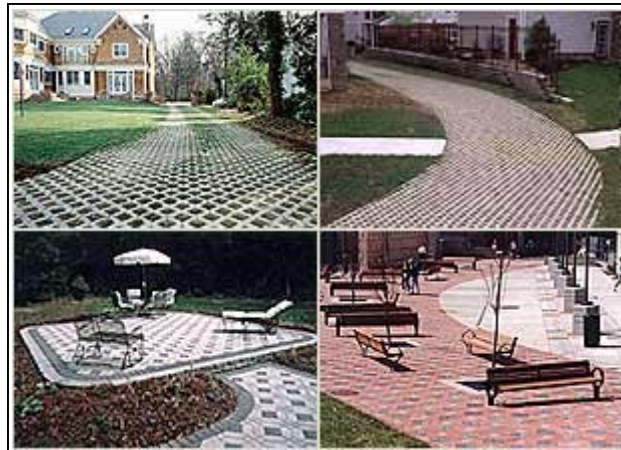
Figure 3.3.8-4 Examples of Porous Paver Surfaces (Sources: Invisible Structures, Inc.; EP Henry Corp.)
